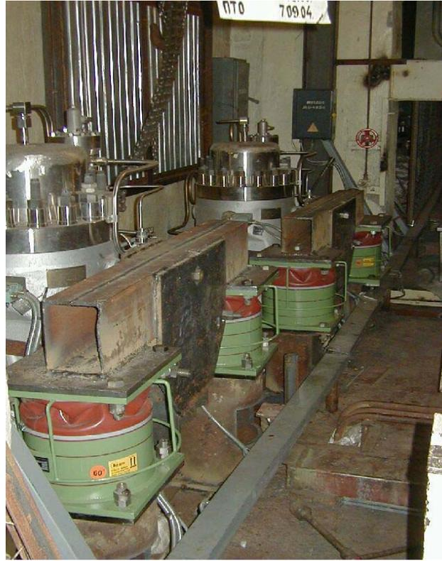
**Figure 7.** General View of the Dampers on the SEBIM Valves 1211 (front) and 1234.
