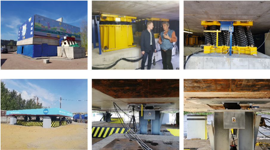
Fig. 11. Upper row: BCS natural scale testing at the Inverse SIST test rig. General View with the variable Superstructure 2 000 tons (left). 3D BCS system with spring units and 3D Viscodamper (middle). Spring Unit under Beyond Design Earthquake Loading (right). Lower row: LRB natural scale testing at the Inverse SIST test rig. General View with the variable Superstructure 400 tons (left). LRBs under full dead weight loading (middle). LRB under seismic displacements (right).
