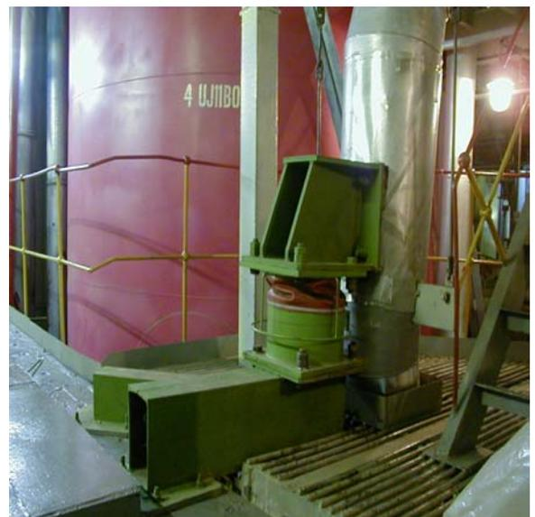
Fig. 13 Installation of GERB Viscous Damper (Run B)
